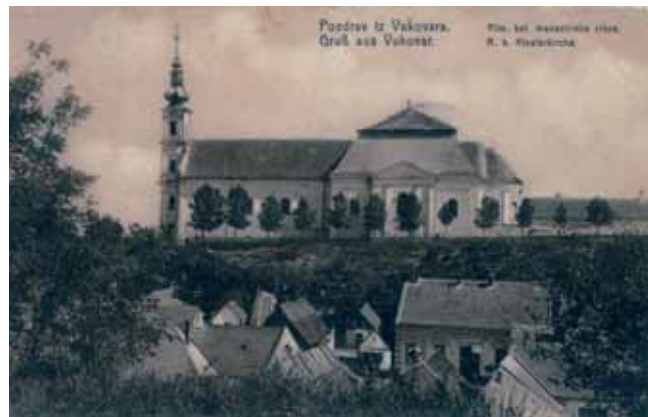
RICHARD JORDAN, FRANJEVAČKA CRKVA U VUKOVARU, PROŠIRENA 1895./ RICHARD JORDAN, FRANCISCAN CHURCH IN VUKOVAR, EXTENDED IN 1895/ RICHARD JORDAN, FRANZISKANERKIRCHE IN VUKOVAR NACH DEM UMBAU, 1895
